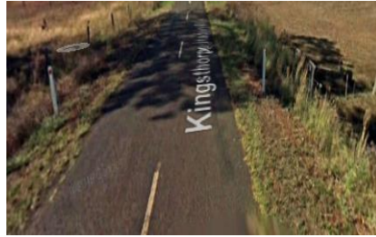
2. Kingsthorpe Haden Road (Culvert)
