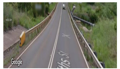
6. Griffiths Street (Bridge)
