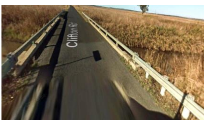
10. Clifton Pittsworth Road (Bridge)
