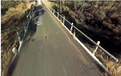
1. Melrose Road (Bridge)
