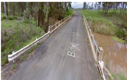
7. Bowenville Moola Road (Bridge)
