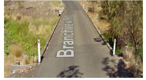
3. Branchview Road (Bridge)
