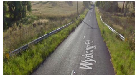
9. Wybong Road (Major Culvert)
