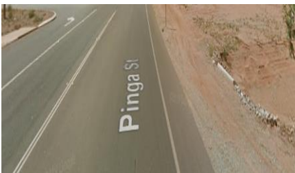
4. Pinga Street Culvert
