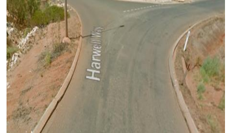
3. Harwell Way Culvert
