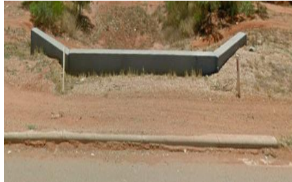
2. North Circular Road Culvert
