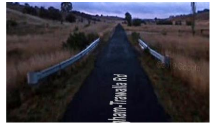
6. Carngham Trawalla Road
