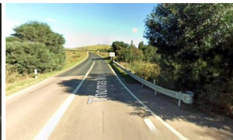
15. Thomas Mitchell Drive (Major Culvert)
