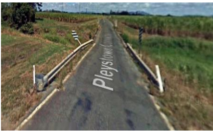
4. Pleystowe Connection Road (Nebia Creek Bridge)
