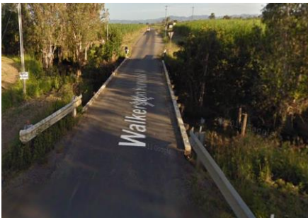
7. Walkerston-Homebush Road (Rocky Creek Bridge)
