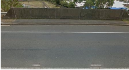
1. Archibald Street Bridge Overpass
