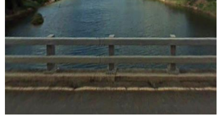
3. Pleystowe Connection Road (John Cook Bridge)
