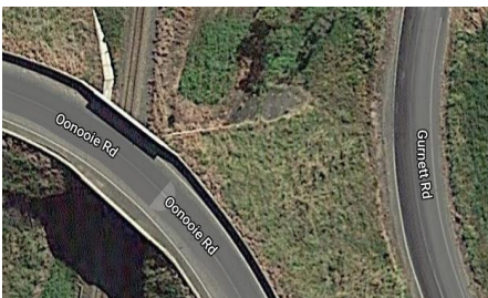
10. Gurnett Rd (Oonoie Rd #2 Overpass)
