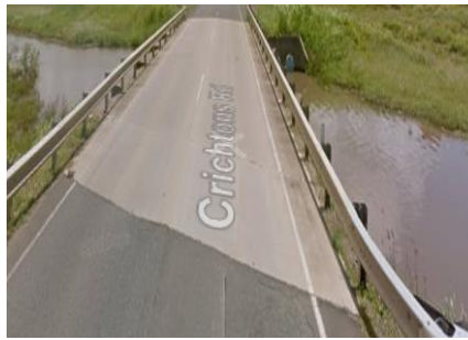
8. Crichtons Road (Major Culvert)
