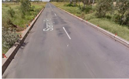
2. Hughes Creek Bridge / Saraji Road
