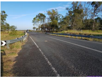
4. Blackburn Creek Bridge / Golden Mile Road
