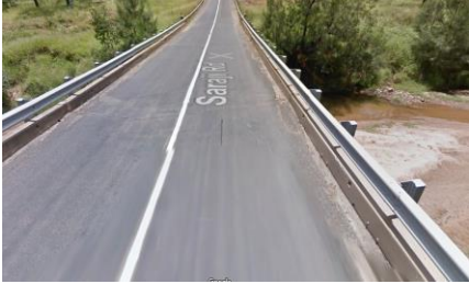
1. Phillips Creek Bridge / Saraji Road
