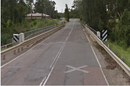
1. Government Road, Kurri Kurri (Homestead Bridge)
