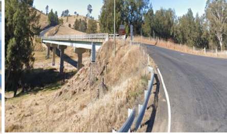
2. Greendale Bridge over Brogo River
